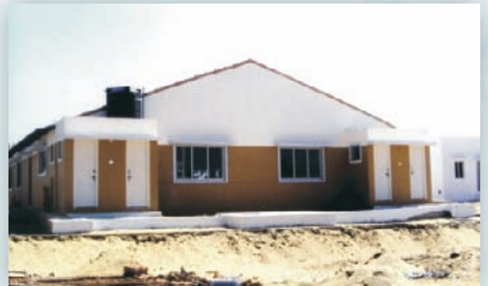
COMMUNITY CENTRE at Kadappakkam Village
